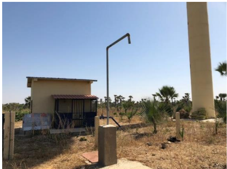
Figure 32 - PUDC Pumping Station for the water tower
